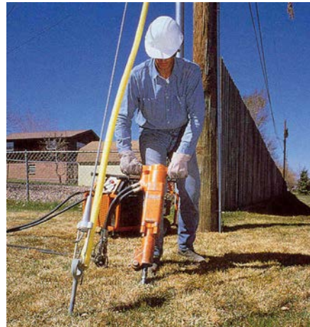
Drive steel coupler at ground level
