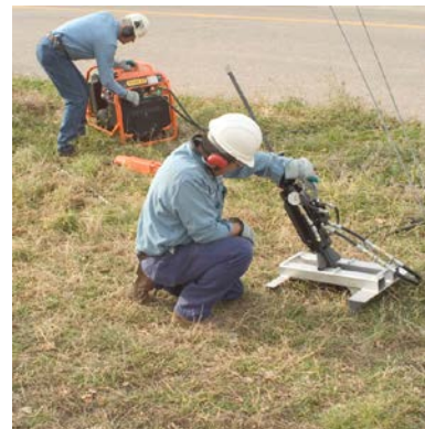
Applying load to the Manta Ray anchor
